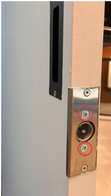
LATCH BOLT ADJUSTMENT
